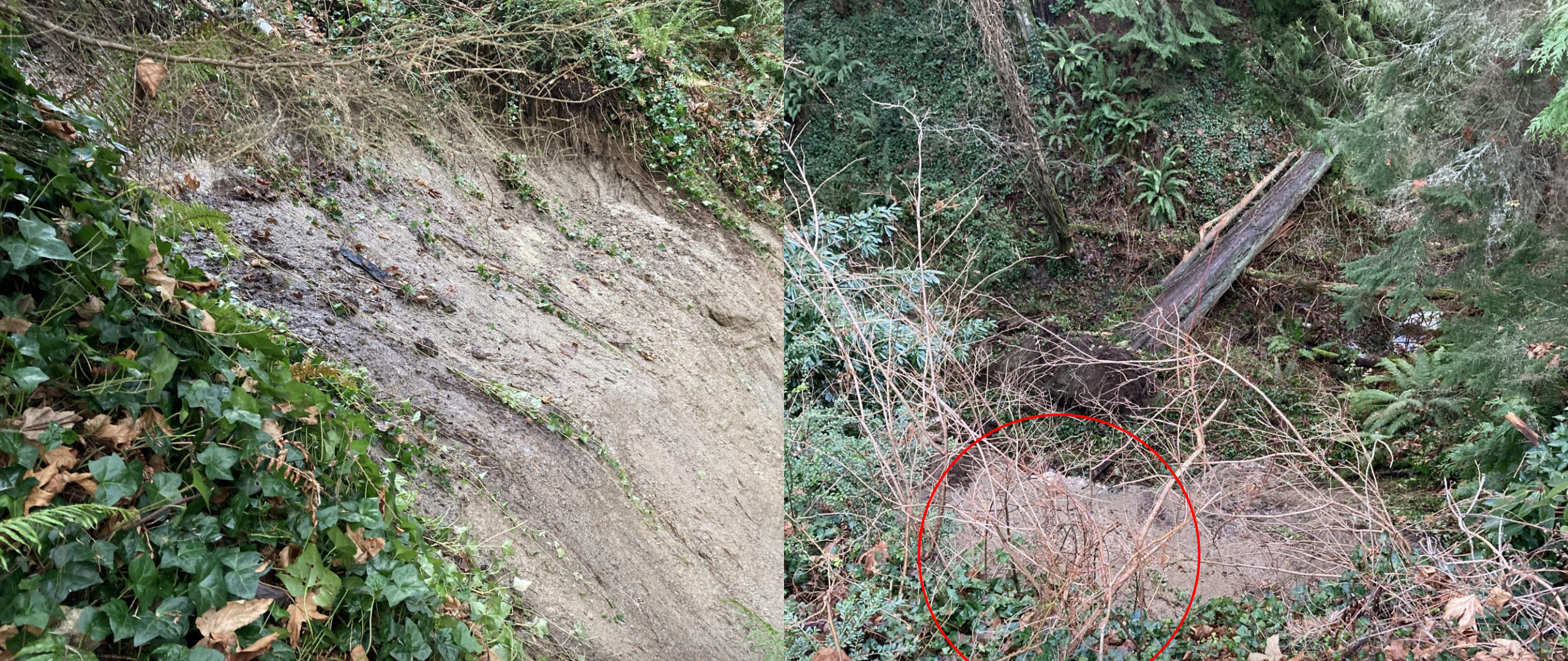
Landslide on Bainbridge Island – duct tapped corrugated pipe
