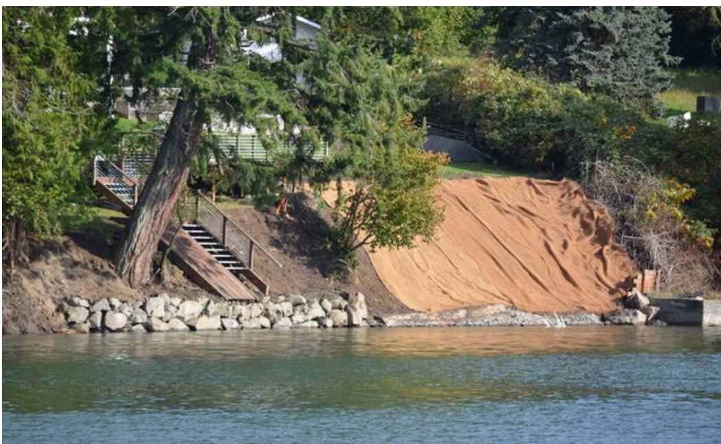
After Construction, October 2019 – Removed section of bulkhead, large wood installation, slope re-contouring and section of replaced bulkhead around access. Photo credit: Jim Haskins
