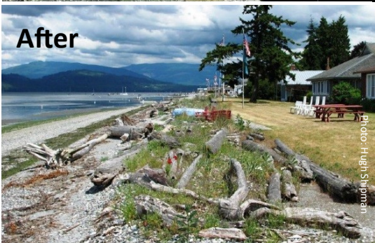
Before and after bulkhead removal and soft shore protection on Samish Island.
